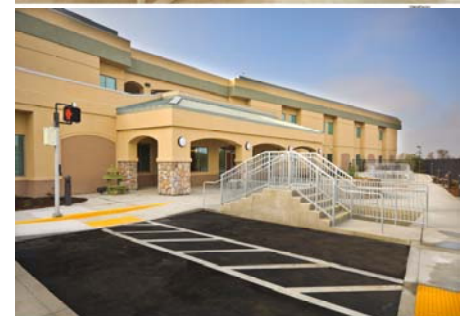
Indoor Rehab Gym and outdoor Multi-Surface Area allows space for physical, and occupational therapists to help patients regain valuable life skills.
